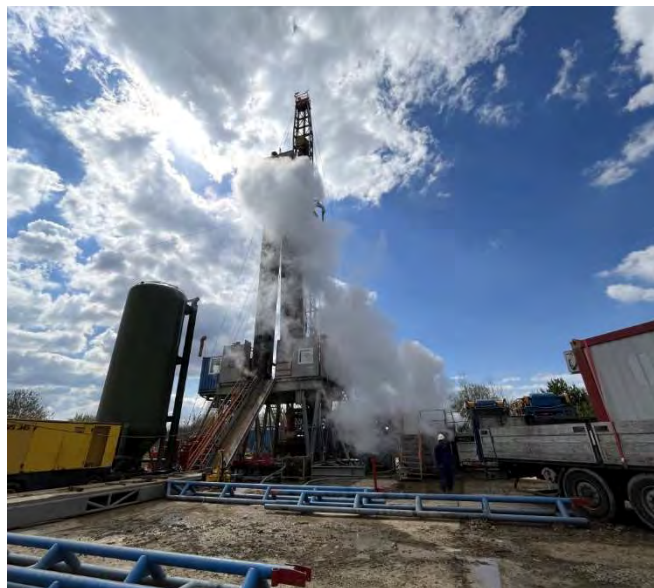
Figure 2: Drilling at the Čížatice site, free-flow with spontaneous steam separation. Photo: Dr. Zuzana Kollová, Dionýz Štúr State institute of Geology – division Košice
