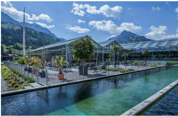
Figure 7: The “Tropenhaus Frutigen” at the northern portal of the Lötschberg base tunnel uses the geothermal heat of the tunnel water for space heating, for raising tropical plants in greenhouses and for producing caviar in a fish farm (source: Tropenhaus Frutigen).
