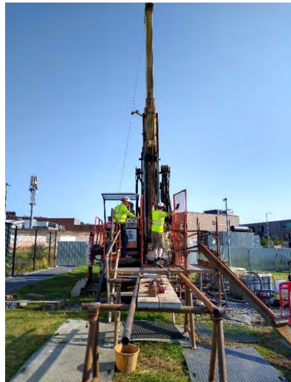
Figure 5: Geological Survey Ireland's drilling rig completing an exploratory borehole at Technological University Dublin, Grangegorman (Photo credit: Sarah Blake).
